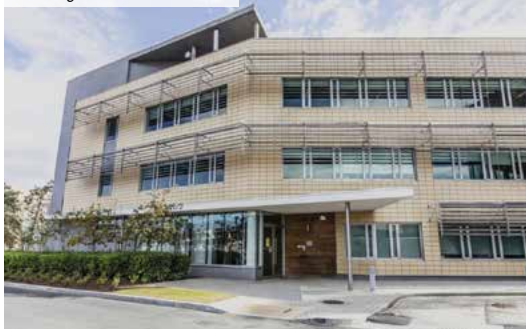
Building 8 – Dublin – Irlande
